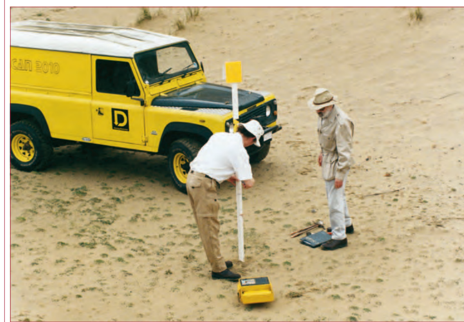
Fig. 3. Making connection to CP test post in Saudi Arabia.
