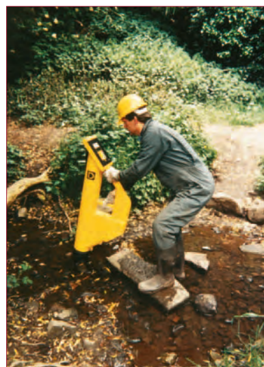
Fig. 1. Survey using a C-Scan 2010 detector unit for a pipeline at a stream crossing.
